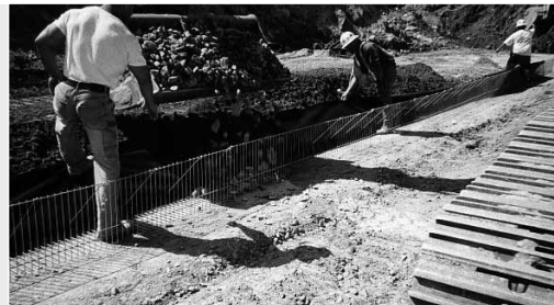
Place stone fill within the Facing Units.
