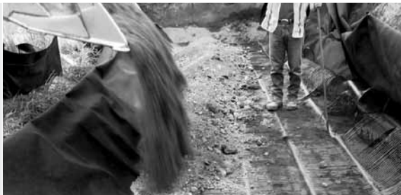
Install backfill over the geotextile separator fabric.
