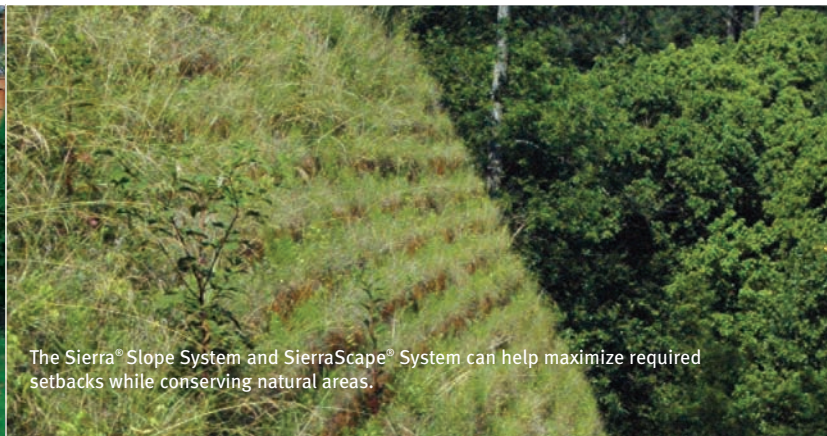
Planting Tensor Grade Separation Solutions with natural vegetative plants helps reduce or eliminate the need for landscape irrigation.
