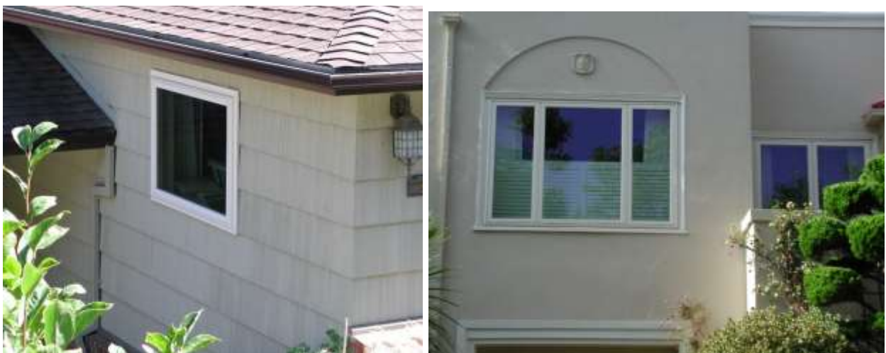
The retrofit replacement windows on a Ranch style house (left) and Spanish Eclectic house (right) provide no reveal.
