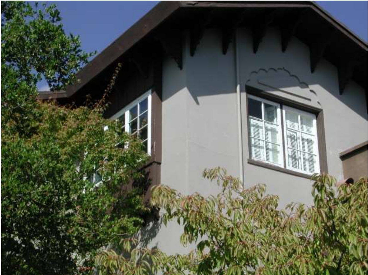
On this Swiss Chalet style house, the window on the right is original and has significant reveal, but the window on the left is a replacement and has no reveal.
