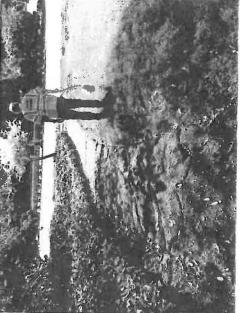
Mature pine tree roots have contributed to uneven paving. With the removal of several large pines, new paving will be less impacted by root damage.
